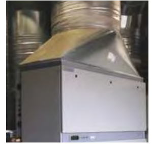
Example of duct installation
